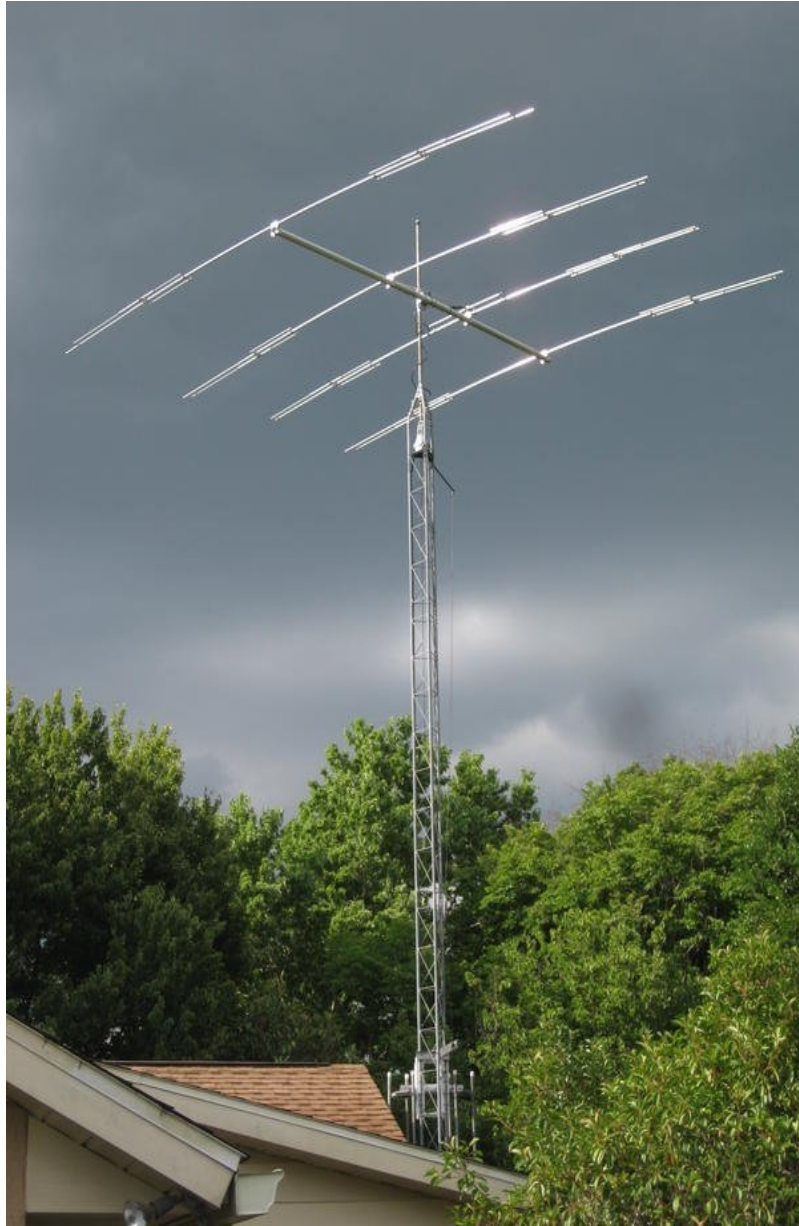
A Beam Antenna on a Tower
